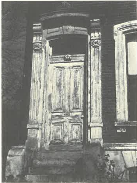
EXAMPLE OF AN EXCELLENT DOORWAY ENTRANCE IN PROSPECT HILL
