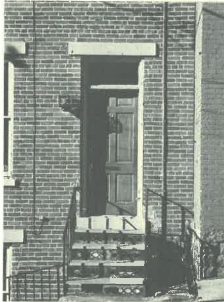
EXAMPLE OF GOOD REPLACEMENT - PANELED WOODEN DOOR IN A RESTORED ENTRANCE
