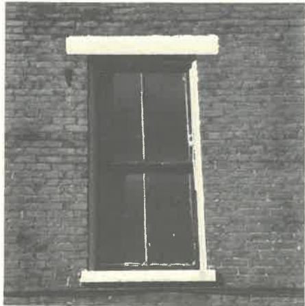
TYPICAL EXISTING "2 OVER 2" WOOD FRAME DOUBLE HUNG FRAME WINDOWS
