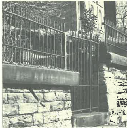
A SIGNIFICANT FEATURE OF THE DISTRICT IS THE IRON FENCES; THESE MUST BE PRESERVED AND ENHANCED
