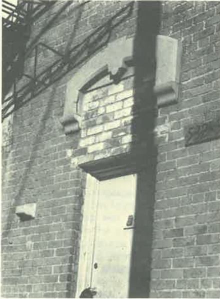
INCORRECT - POORLY DONE REPLACEMENT DOOR (FLUSH MODERN DOOR AND REMOVAL OF TRANSOM WINDOW)
